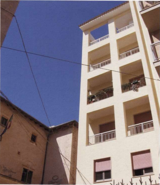
4.5 - Via Gargallo, condominio
